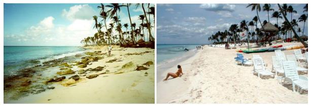
Figure 5. Increased Beach Width 1998 to 2001 at Center of Project - looking west.
