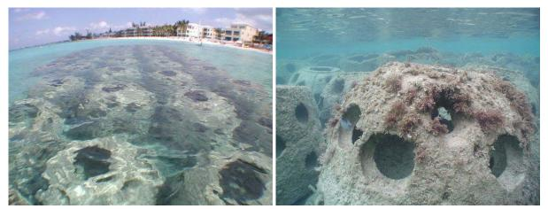
Figure 6. Photographs of 5-Row Reef Ball Breakwater offshore Grand Cayman
