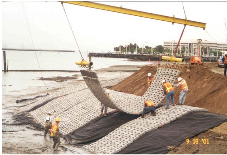
Figure 3-6. Installation of ABM's using a spreader bar (URS, 2001).
