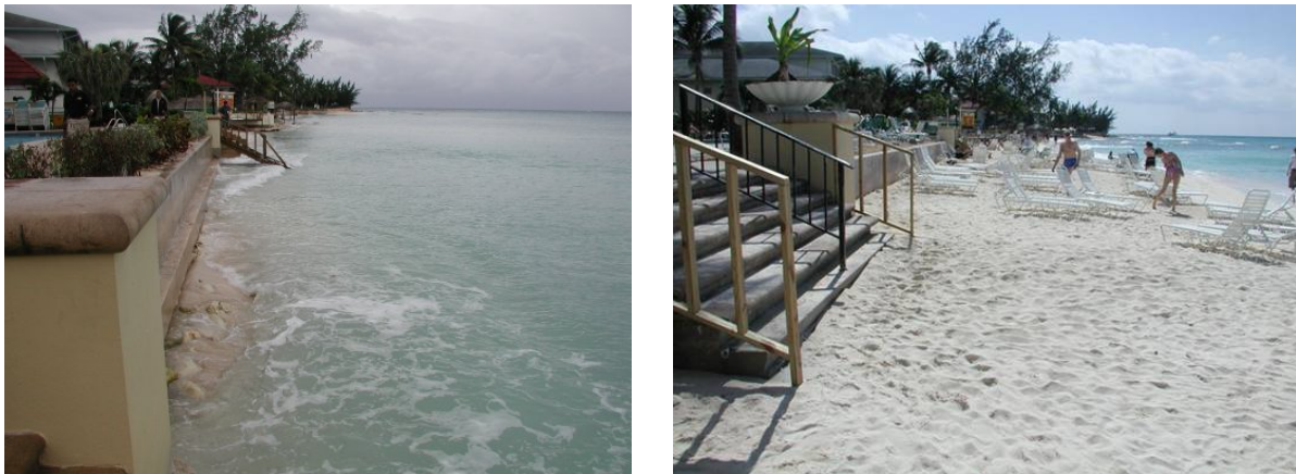
Figure 8. Marriott Beach Before (L) and After (R) Reef Ball Breakwater Installation
