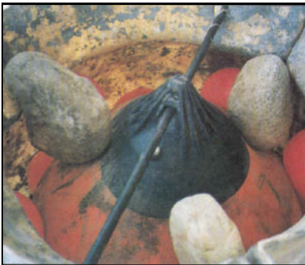
REEFBALLS: Inflatable bouys give shape to the concrete tunnels (left); and a finished ball (right)
